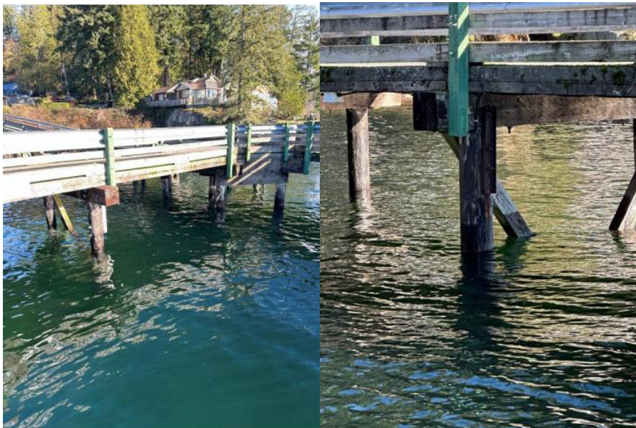
Figure 2-1 Gambier Harbour – Typical arrangement of timber piles
