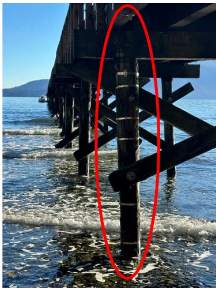
Figure 12. West Bay Pile 6A – to be tested
