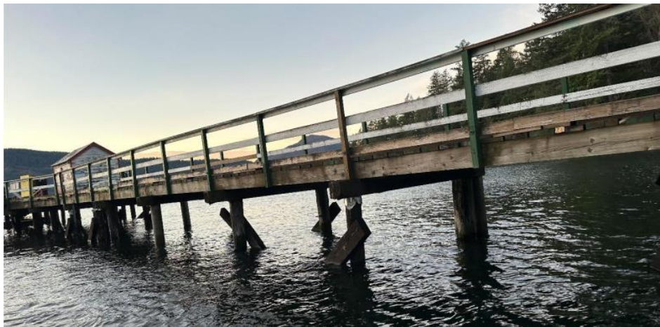
Figure 15. Halkett Bay – Overall View of the facility
