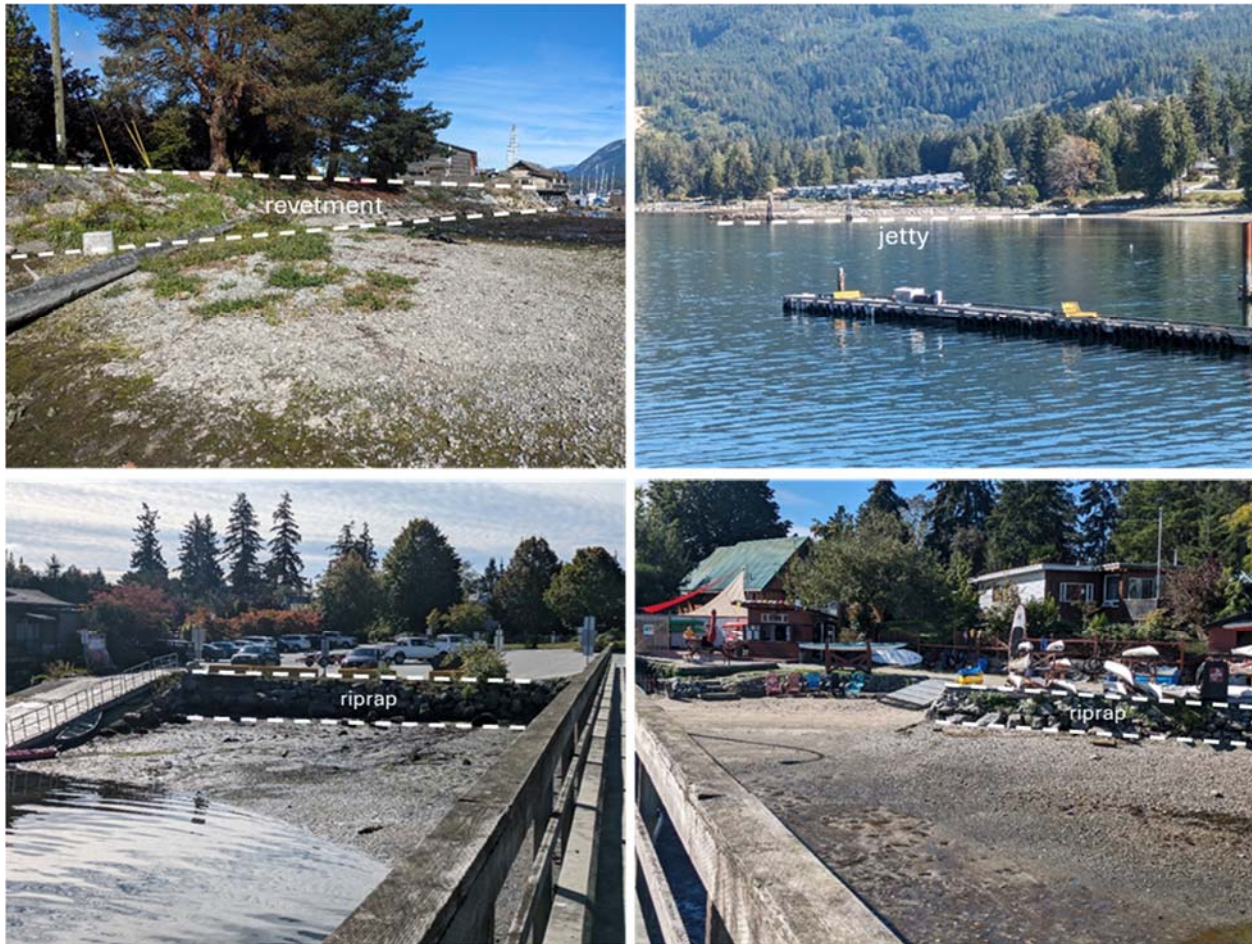
Photo 3 Shoreline protection features on the southern shoreline of Sechelt Inlet.
