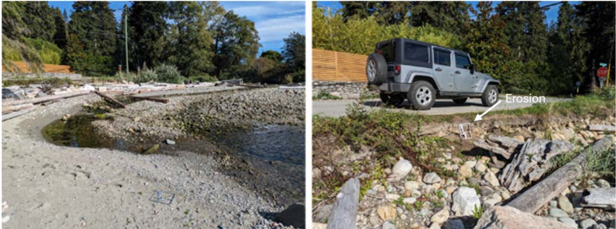
Photo 7 Chaster Creek northern outlet channel (left) and shoreline erosion (right).
