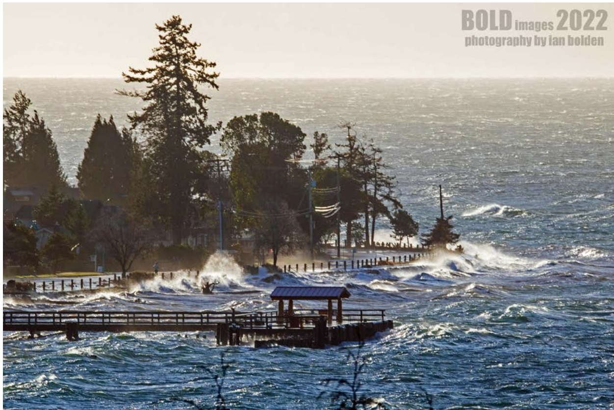
Figure 1.2 Wave overtopping near Davis Bay during a storm event (January 7, 2022). Elevated water levels and wave run-up caused localized flooding along Sunshine Coast Highway (source: Ian Pipes Bolden).
