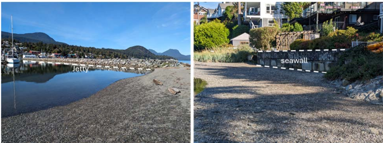
Photo 8 Gibsons Bay shoreline protection features near Bay Road.
