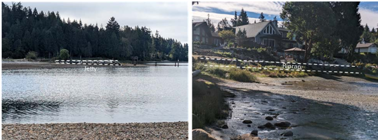
Photo 2 Shoreline protection features observed near Marmot Road.
