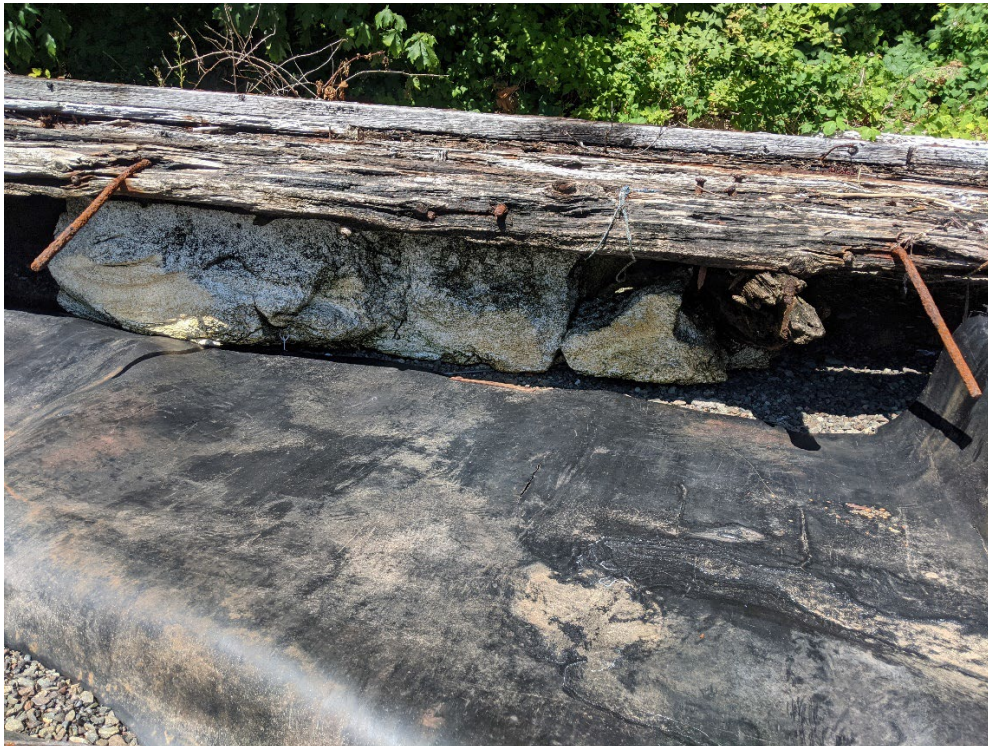
Figure 3- Goliath Bay, Expanded Polystyrene (EPS) (Styrofoam) and HDPE Plastic Sheetting
