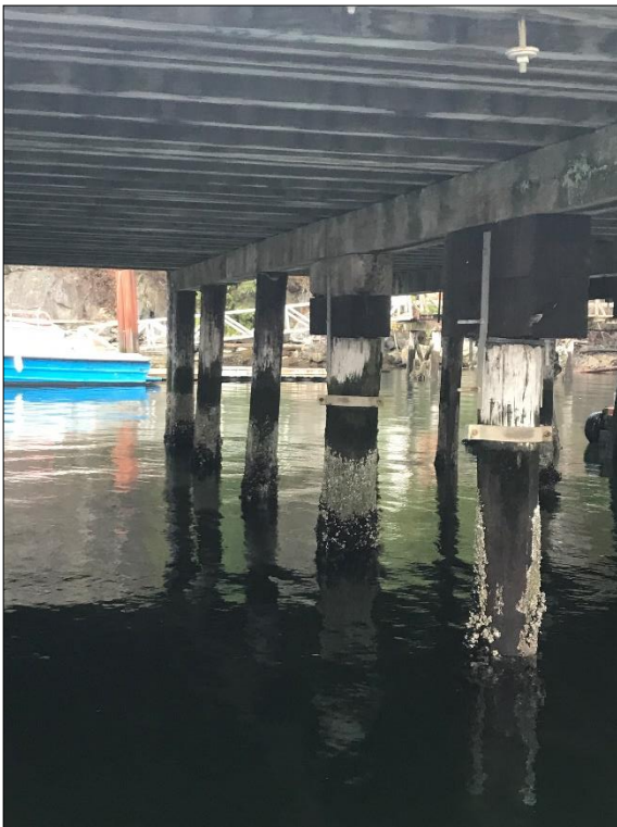
Photograph 6: Bearing pile repairs, note: strap does not extend to pilecap
