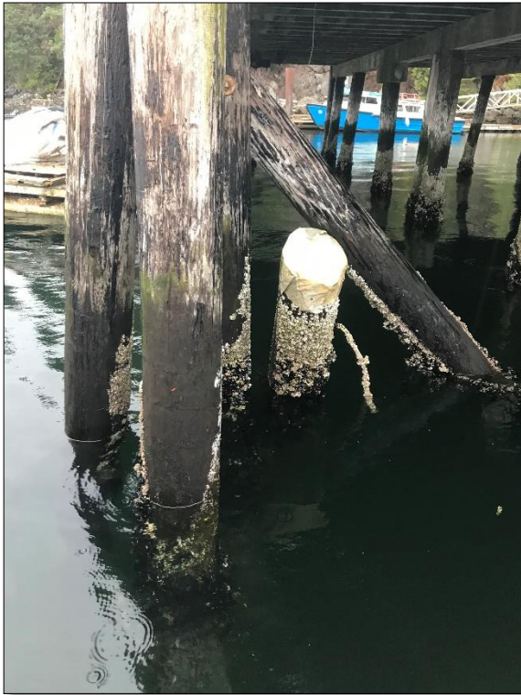
Photograph 7: Batter pile 20A east to west, note: no longer connected to bearing pile
