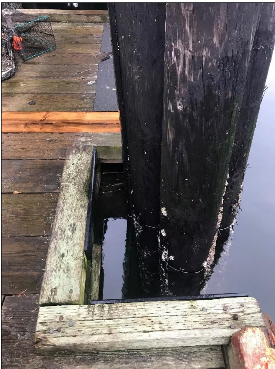
Photograph 14: Mooring pile well, note: not restraining mooring piles
