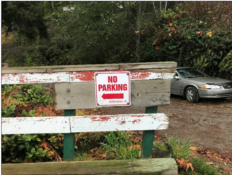
Photograph 2: Approach handrails and guard, note: deterioration due to weathering and biological damage
