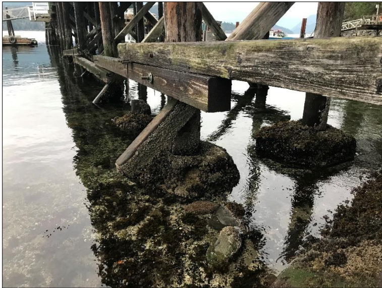
Photograph 4: Bearing pile 5A, note: spalling of the concrete footing
