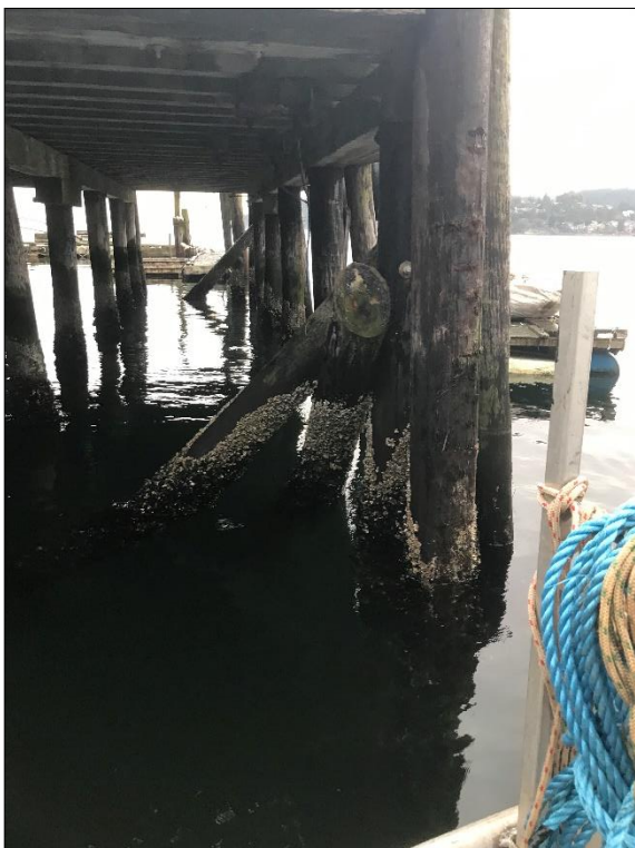
Photograph 8: Batter pile 20F, note: no aluminum flashing at cut end
