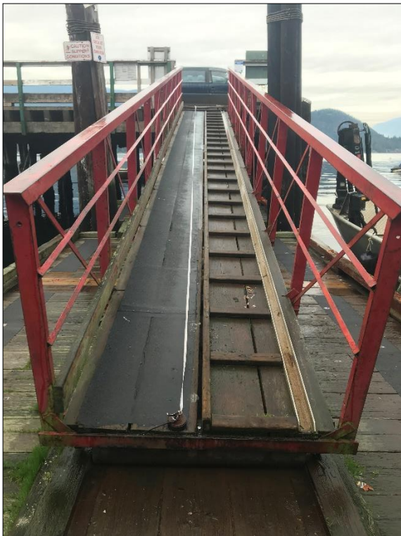
Photograph 12: Gangway, note: minor coating losses and surface corrosion of the steel
