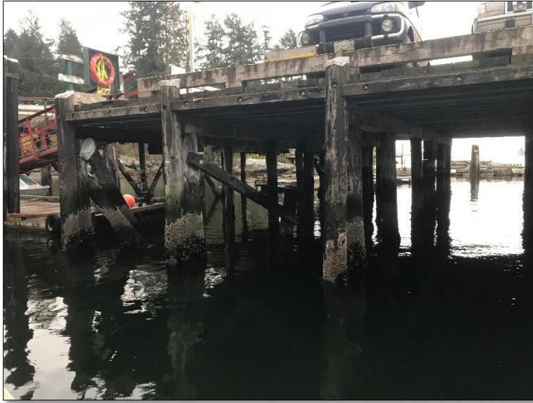
Photograph 17: Miscellaneous bracing connected to abandoned piling, note: potential navigation hazard
