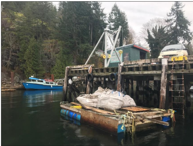
Photograph 18: Miscellaneous scow with debris secured to wharf, note: insufficient fendering for this application
