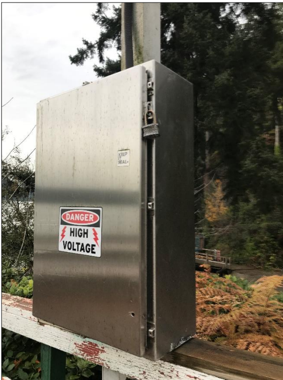
Photograph 16: Electrical service box, note: no lock at bottom connection
