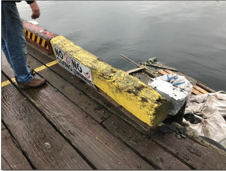
Photograph 5: Guard on wharfhead, note: to be replaced
