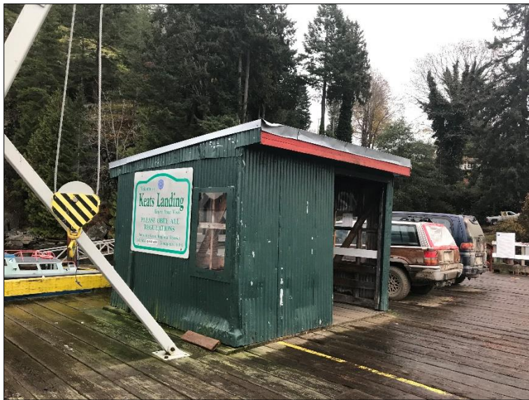
Photograph 10: Service shed, note: mechanical damage to siding
