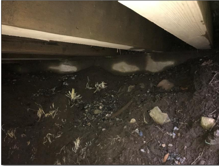
Photograph 3: Concrete abutment, note: water seepage
