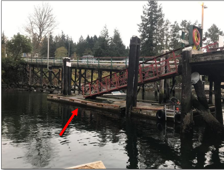
Photograph 13: Float, note: low point at gangway roller
