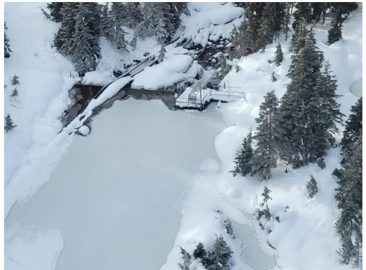
Channel and dam at Chapman Lake January 30, 2023
