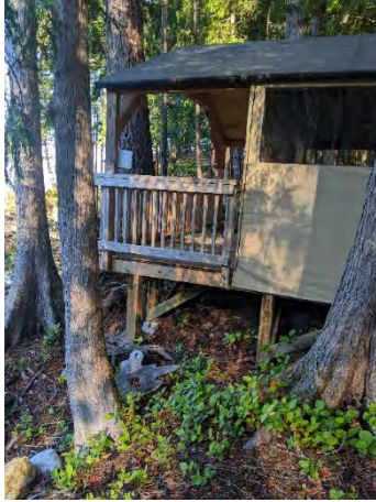
View of the structure and proximity to adjacent trees.
