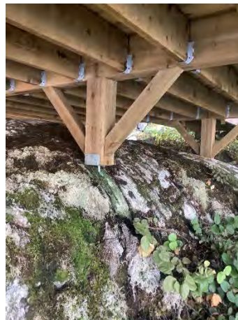
View of understory and footings beneath the building and deck.
