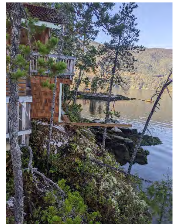
View of the building and the raised rockface cliff.
