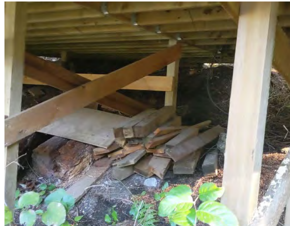
View of beneath the deck.
