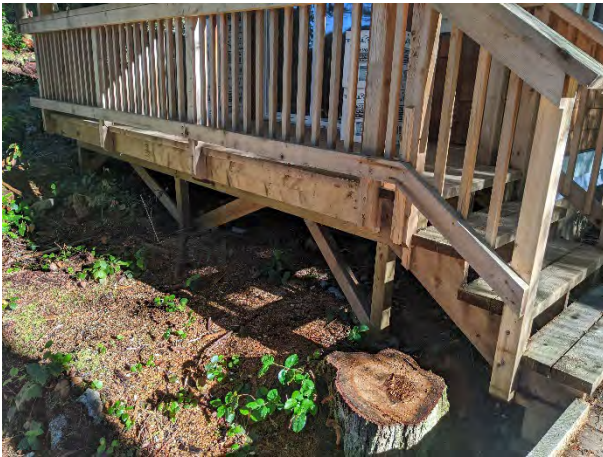
View of footings and understory disturbance around building 3.
