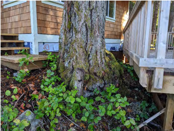
Building 4 and a deck has been built around a large Douglas-fir.
