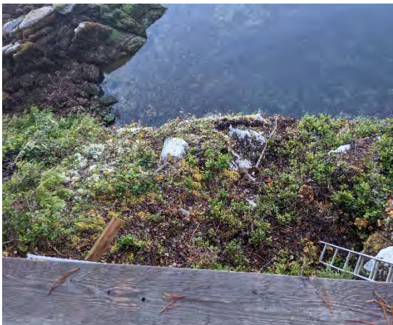
View of the horizontal distance between the deck edge and the water.
