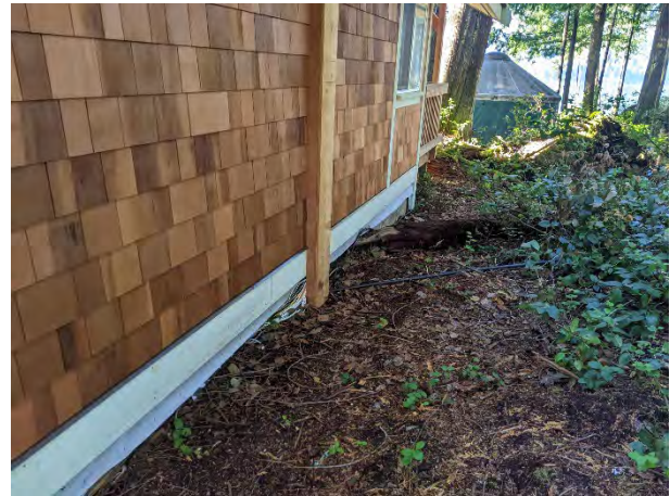
View of understory disturbance around building 3.
