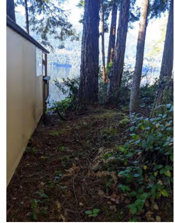
View of the understory brushing around the structure.
