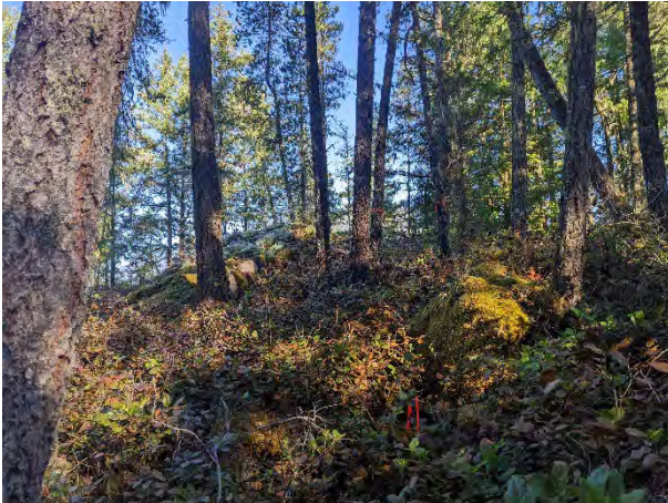
View of orange flagging along the planned boardwalk access to building 10.
