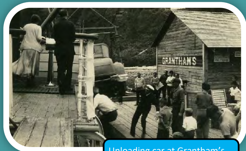
Unloading car at Grantham's, 1930s Photo # 2406
