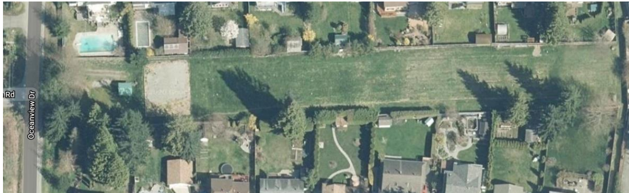
Figure 1 - WWTP and Disposal Aerial View
