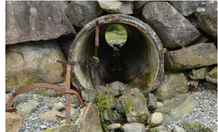
Existing condition of culvert at foreshore and Fisherman Road.
