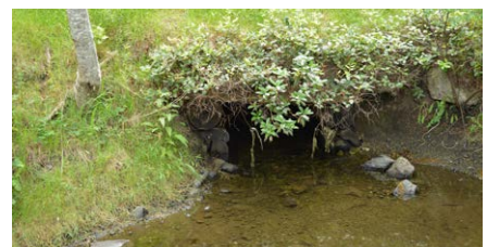
Existing condition of box culvert at pond and Redrooffs Road.
