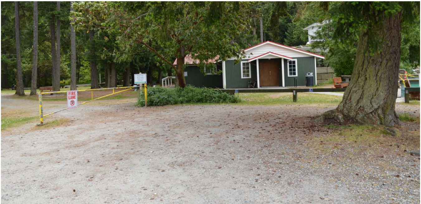
View to existing Community Hall from Fisherman Road end.
