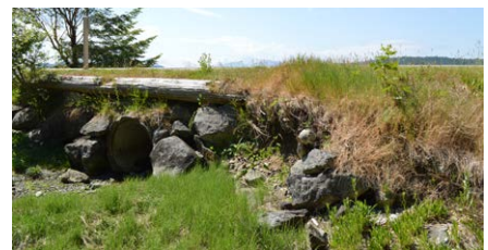
Existing condition of culvert and headwall at pond and Fisherman Road.
