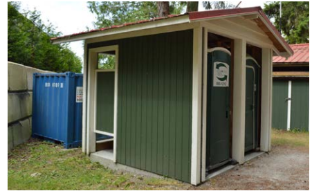
Existing outdoor washroom building with portable toilets and changeroom stalls is located in close proximity to property line, adjacent to lock block concrete retaining wall.
