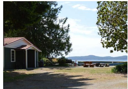
The existing Community Hall was built in the 1980s and is non-conforming with setback requirements.
