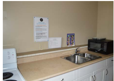
The current kitchen facility cannot support efficient catering for large groups.
