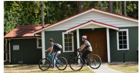
Current on-site amenities for bikes are limited to one bike rack by the existing hall entrance.
