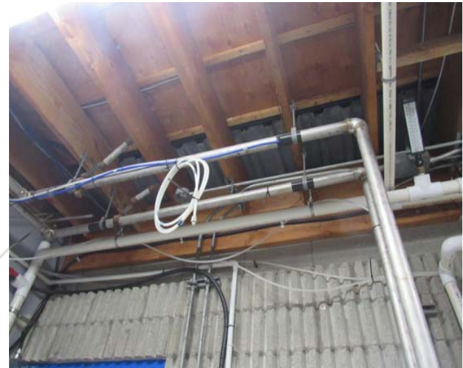
Photo #S2: Wood framing at extension section in northwest corner of the building.
