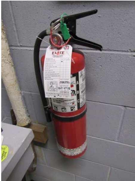
Photo #M9: ABC type fire extinguishers provided throughout.
