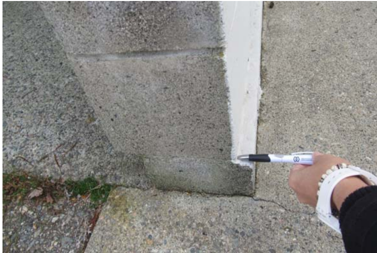
Photo #S7: No dowels provided to between wall and foundation wall.
