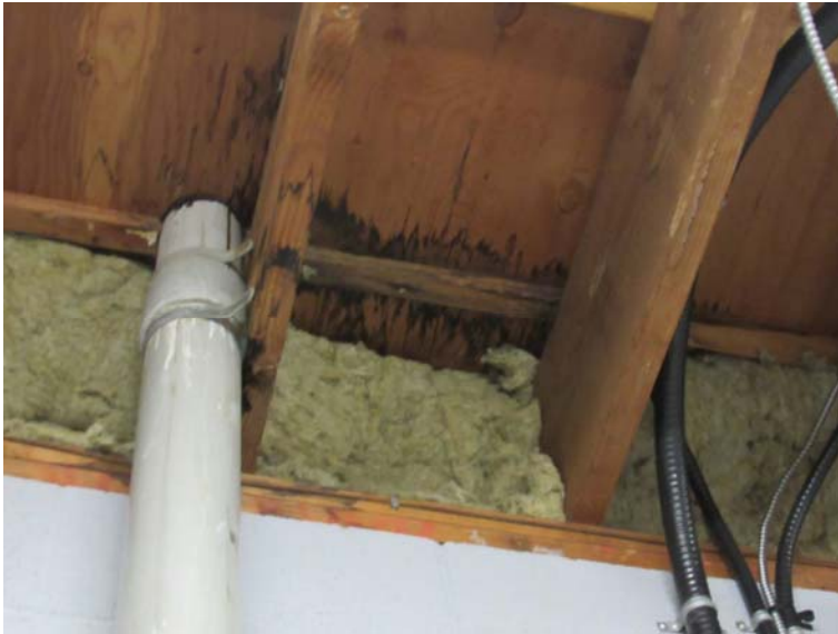
Photo #S3: Localized water stains in wood roof structure.
