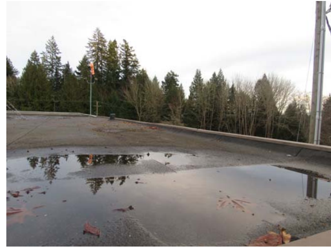
Photo #A18: Ponding observed on the SBS roof on the south building section.
