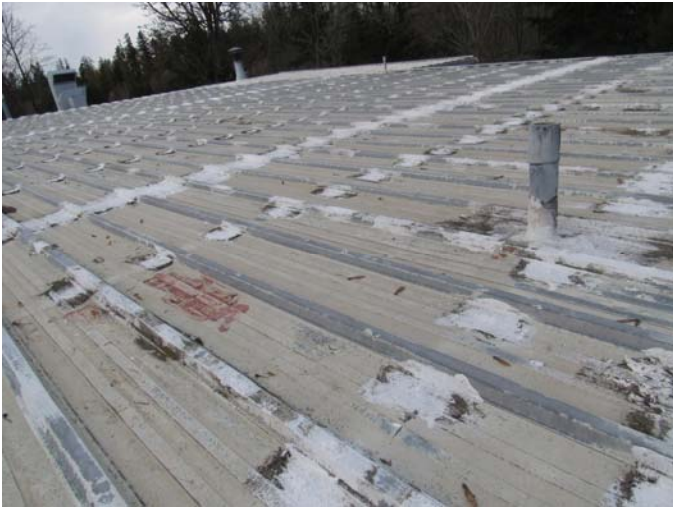
Photo #A17: Typical condition of the main standing metal seam roof.
