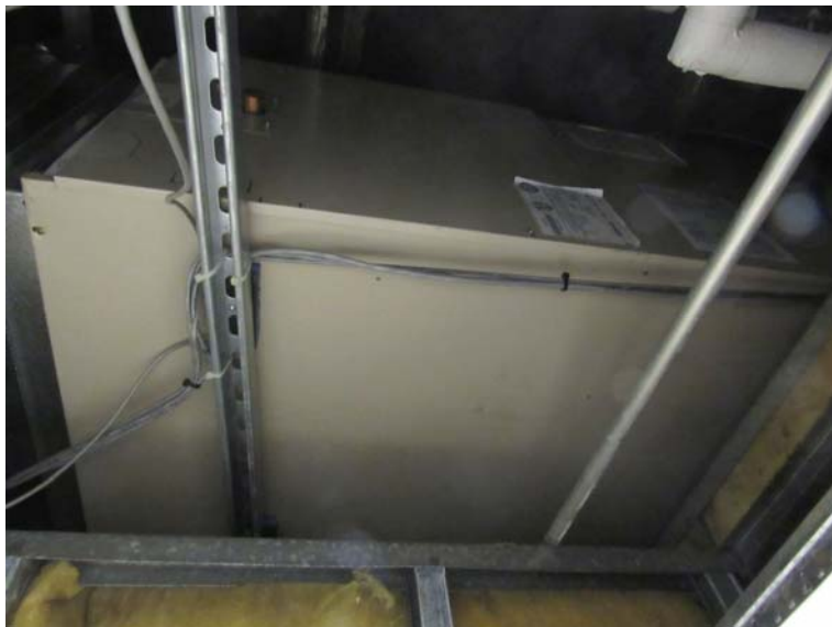
Photo #M7: Air handling unit within the ceiling space.
