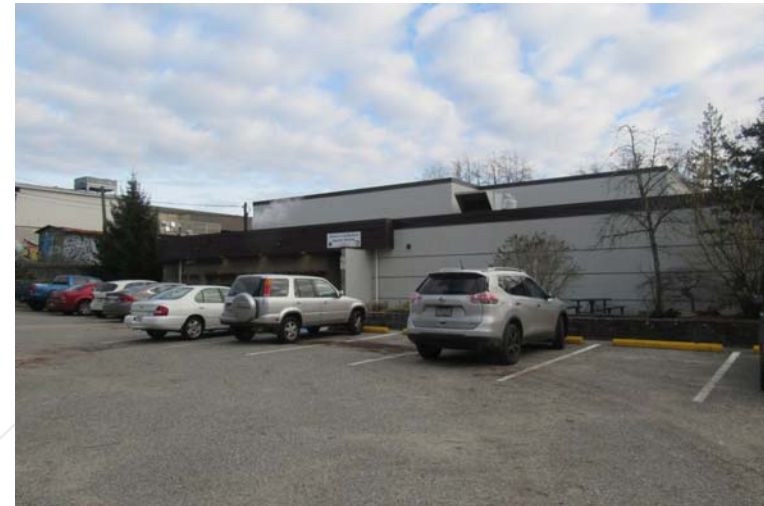
Photo #A6: Overview of front elevation of the building. Typical exterior CMU walls EIFS and cladding finish.
