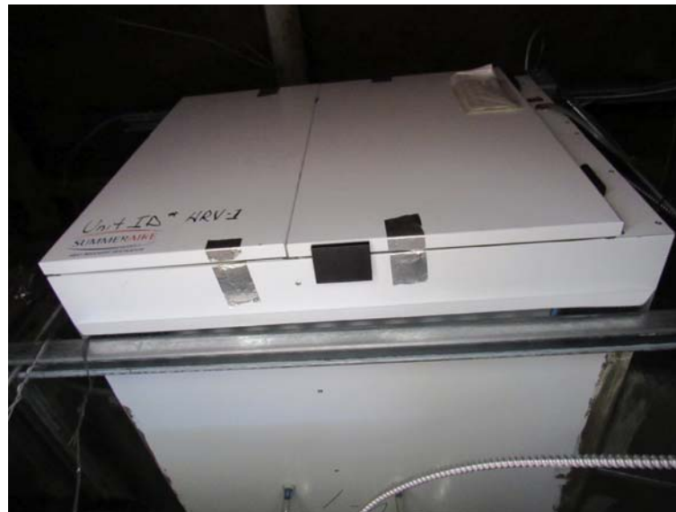
Photo #M8: HRV within the ceiling space.
