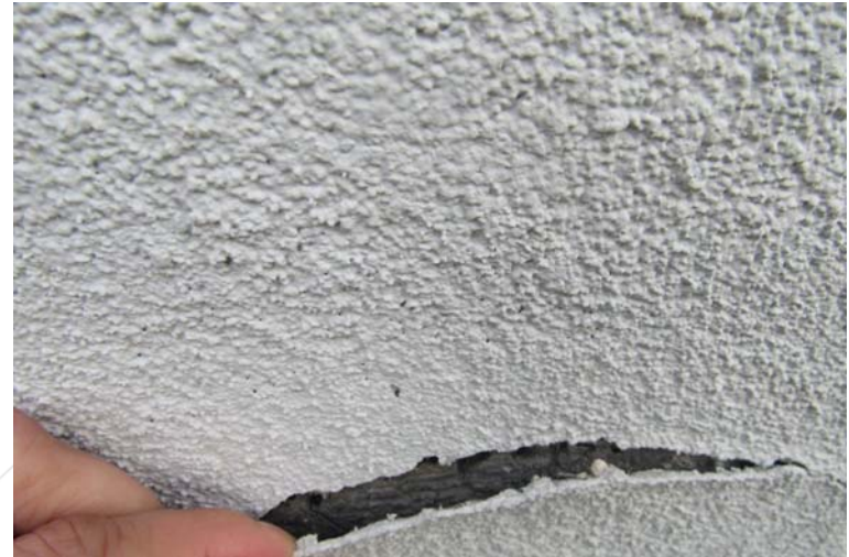
Photo #A8: Deterioration observed EIFS cladding finish.
