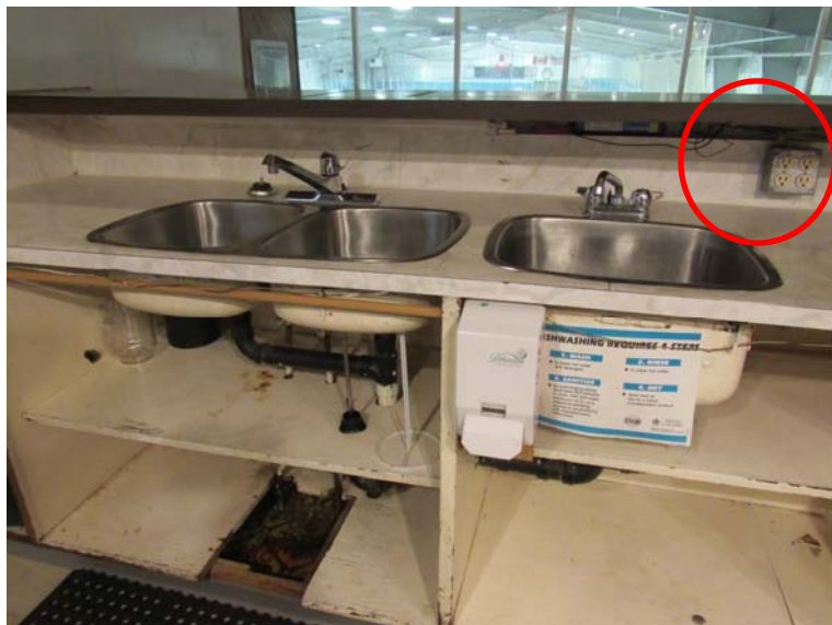
Photo #E5: Missing GFCI receptacle near sink.
