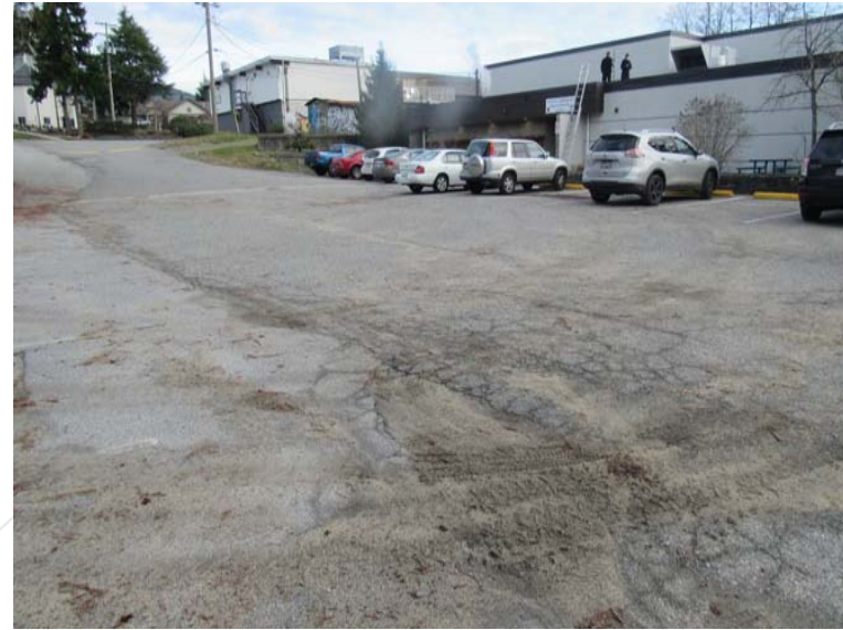
Photo #A2: Some alligator cracking at northwest side of the site.
