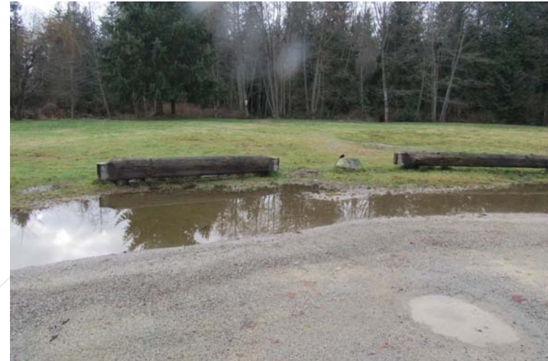
Photo #A4: Observed water ponding at south side of site.
