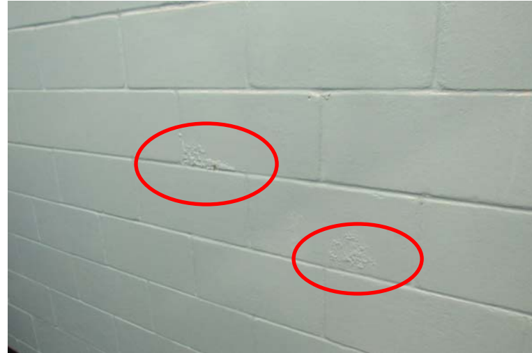
Photo #S6: Signs of moisture on the north wall at the west building addition.
