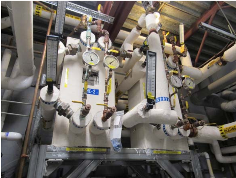
Photo #M3: Two of the three (3) heat exchangers observed on site.
