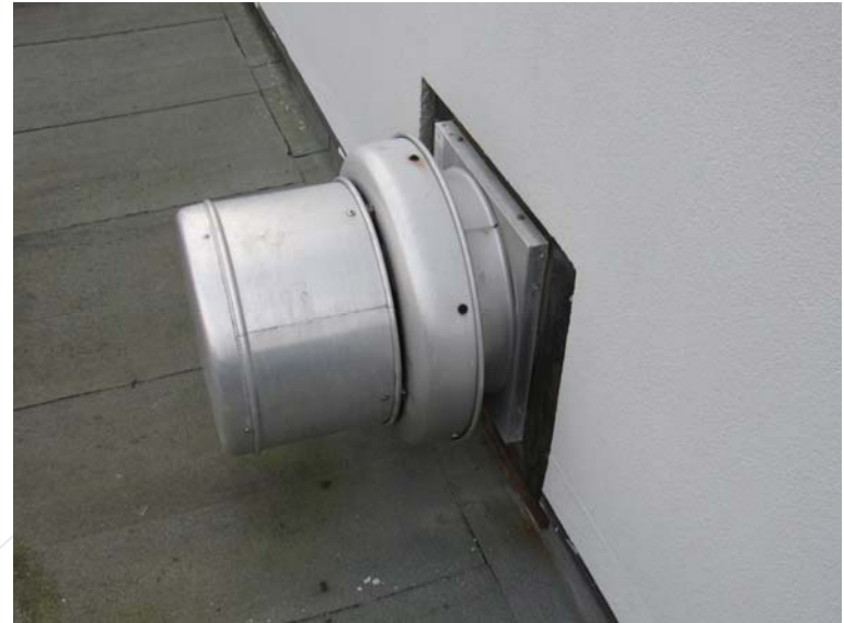
Photo #M8: Dome type wall mounted exhaust fan for natatorium area.
