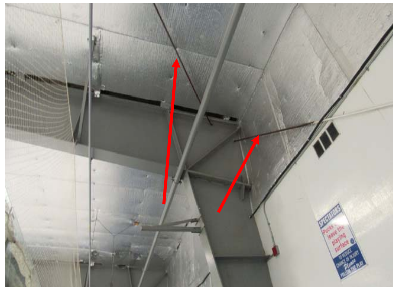
Photo #S4: Some of the corrosion observed on the cross-bracing members.
