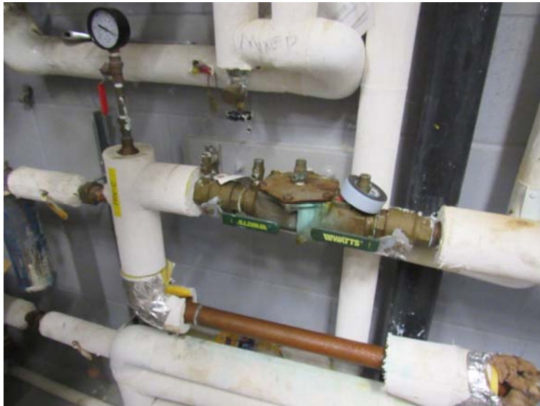
Photo #M1: One of the three (3) backflow preventers observed on site.
