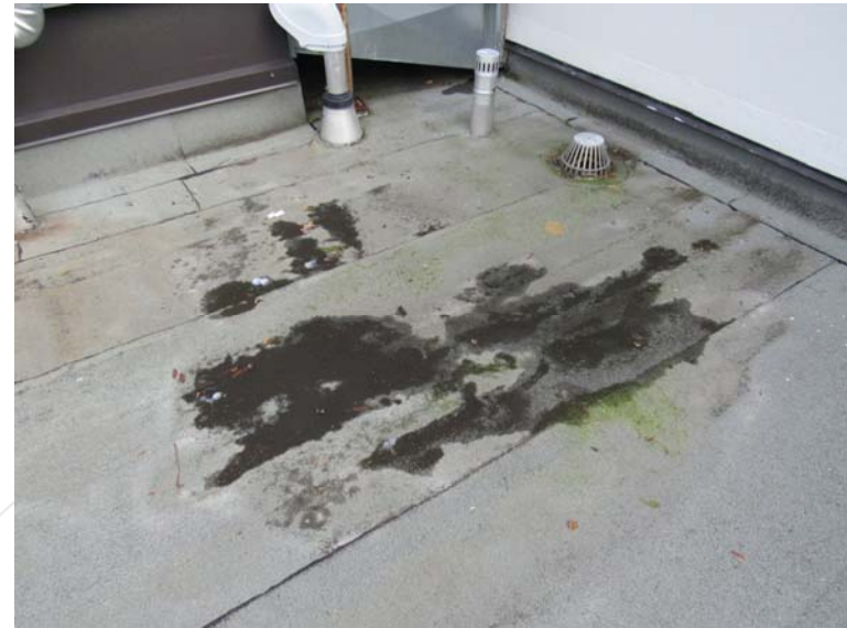
Photo #A18: Sign of ponding observed on the SBS roof.
