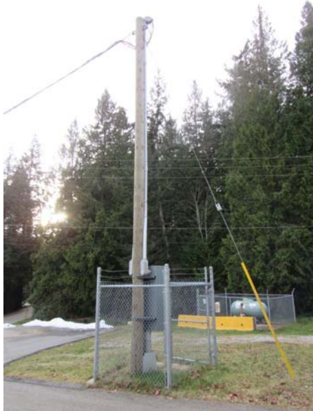
Photo #E1: Electrical service conductors.
