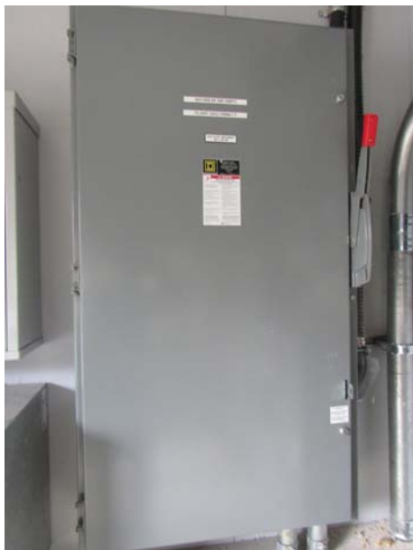
Photo #E3: Main disconnect switch.
