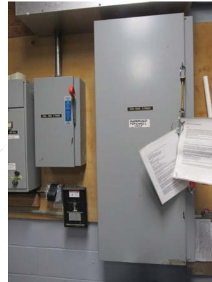
Photo #E2: Main disconnect switch equipment in the mechanical room.
