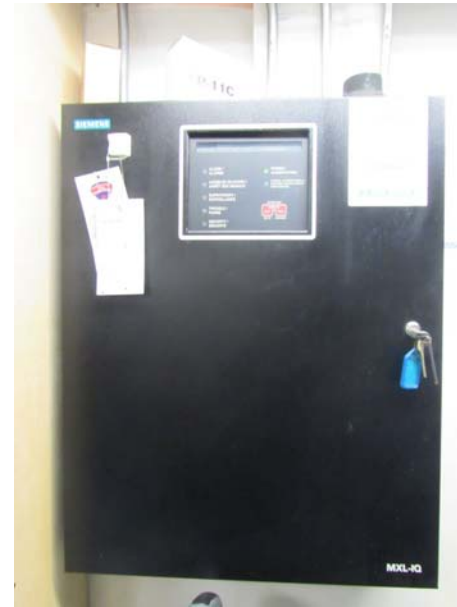
Photo #E10: Fire alarm panel in the sprinkler room.
