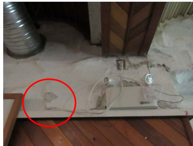
Photo #A16: Friable asbestos plaster in the lounge.
