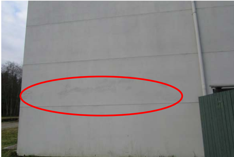
Photo #A7: Sign of water infiltration on EIFS cladding finish.
