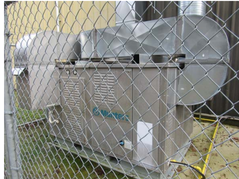
Photo #M10: Outdoor dehumidifier unit serving the arena.
