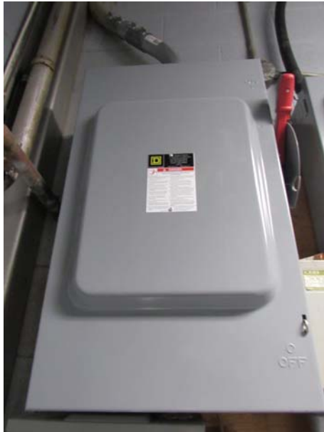
Photo #E3: Main disconnect switch in electrical room.
