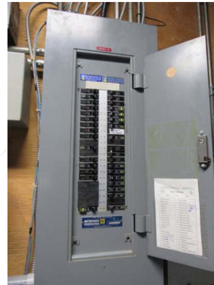
Photo #E4: Typical secondary distribution panel.
