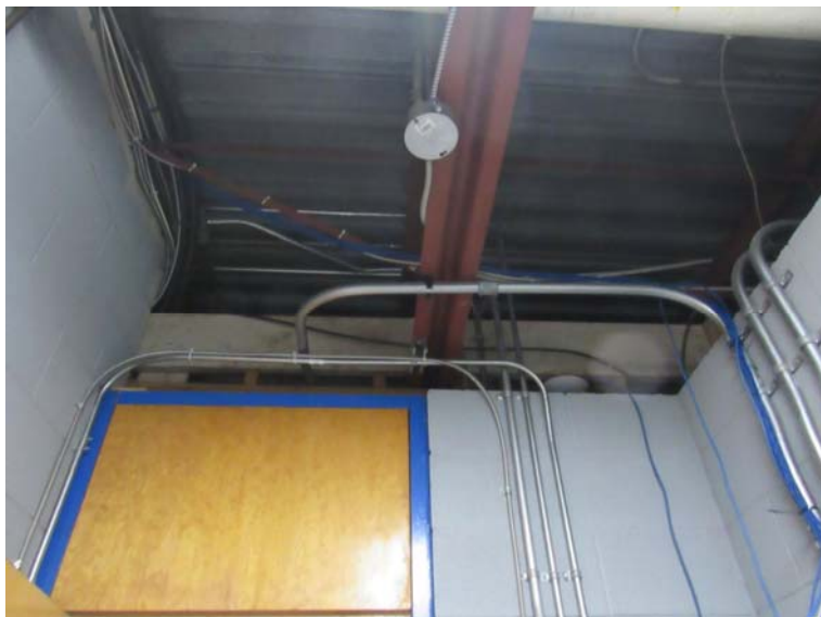
Photo #E5: Missing fire stopping sealants in electrical room.
