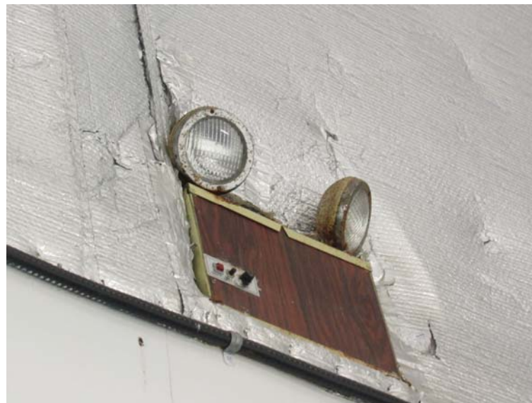
Photo #E8: Original emergency battery packs in the arena.
