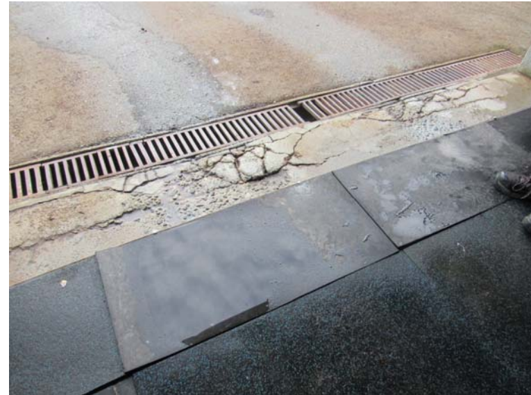
Photo #A4: Observed condition of the trench drain and concrete at the Zamboni Room exterior door.
