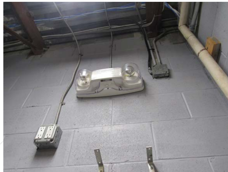
Photo #E8: Emergency battery packs throughout.
