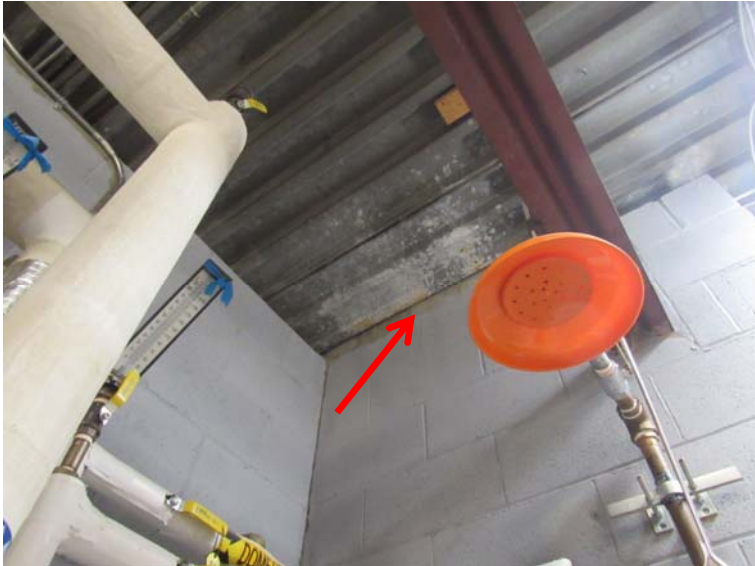
Photo #A19: Sign of water infiltration from the roof (mechanical room).
