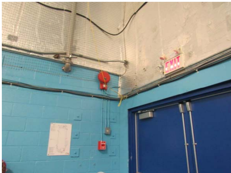
Photo #E7: Exit lighting and some fire alarm devices.
