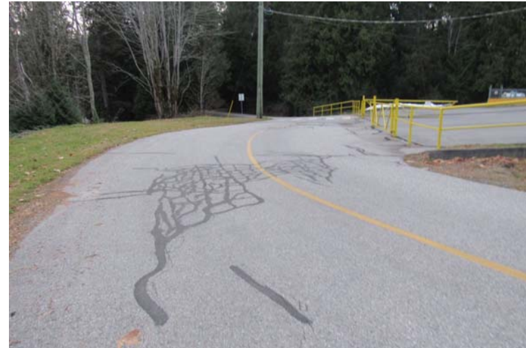
Photo #A2: Some crack pavement repairs noted on the access road to the parking lot.
