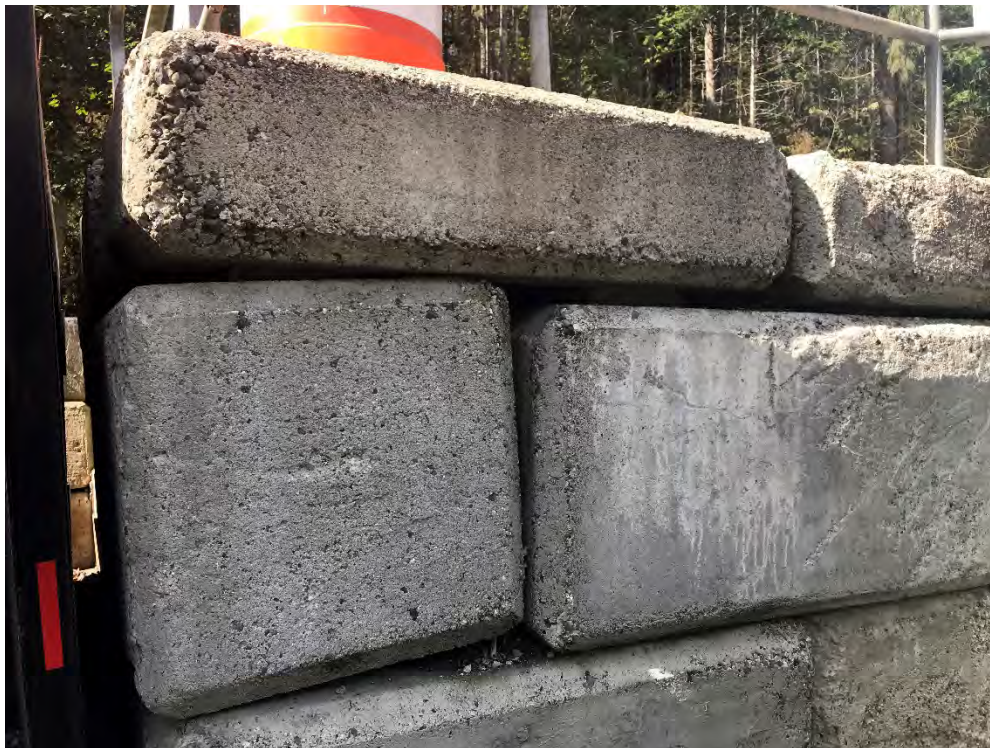
Photograph 10: Uneven lock block at open wall locations.
