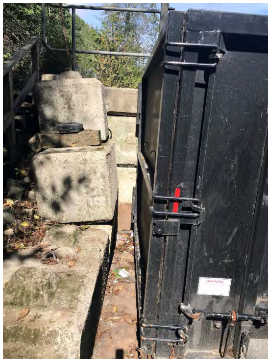
Photograph 12: Uneven lock block at the drop off area stairs.
