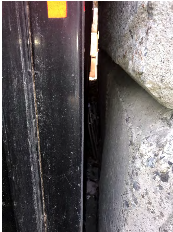
Photograph 9: Uneven lock blocks behind 40-yard bins.
