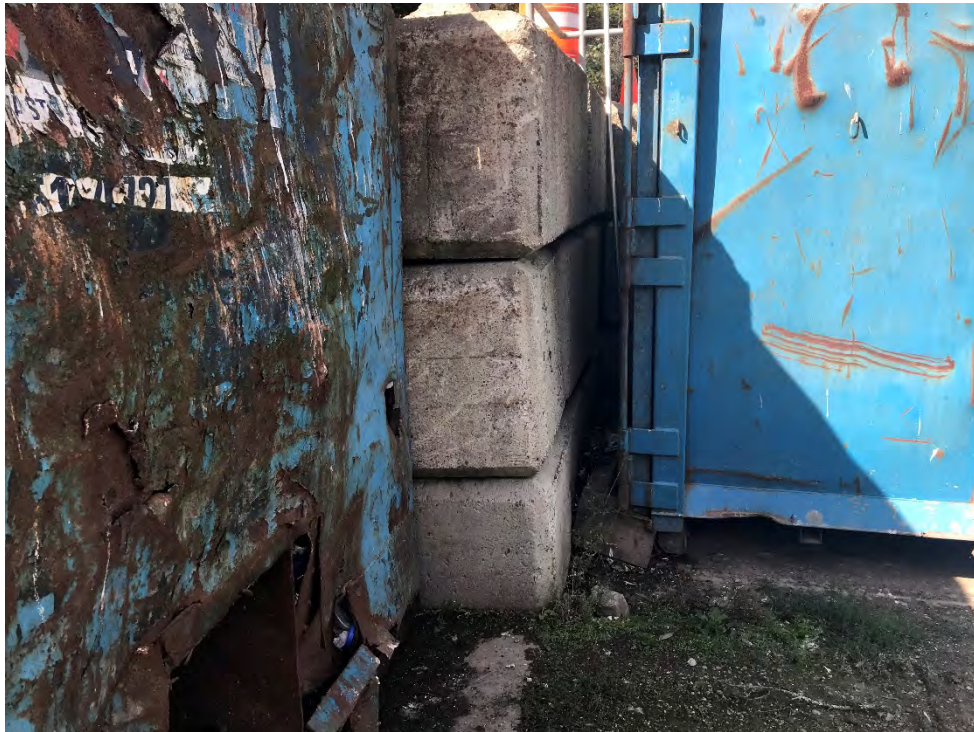
Photograph 11: Uneven lock blocks at corner of lock block wall.
