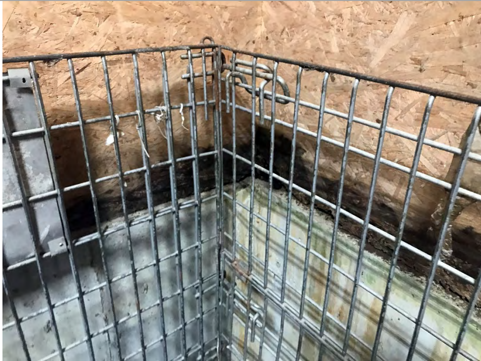
Photograph 15: Interior share shed wall showing signs of excess water rot.
