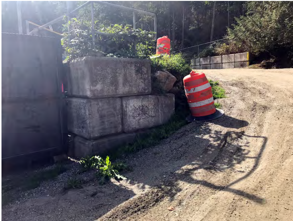
Photograph 7: Drainage at the end of lock block wall.
