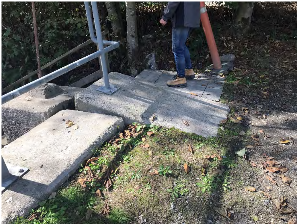
Photograph 8: Lock block wall issues at drop off area stairs.
