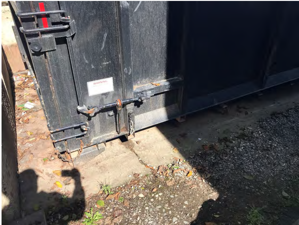
Photograph 13: Cracked concrete bin pad.
