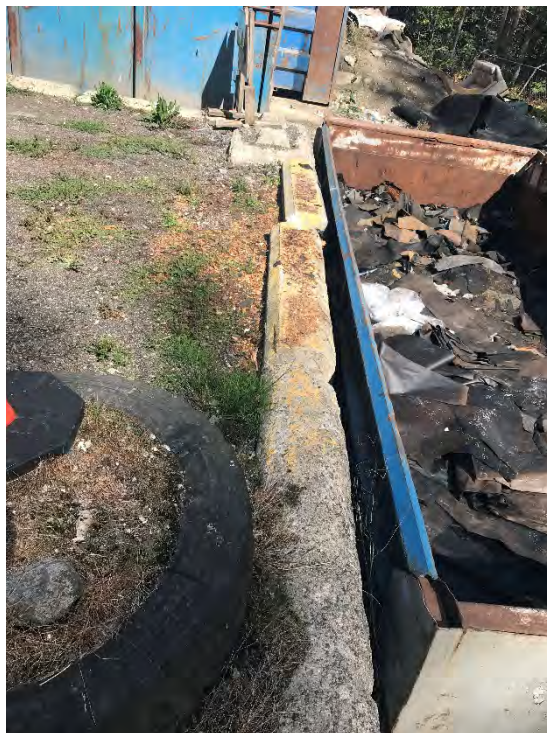
Photograph 14: Uneven lock blocks at the cardboard bins.
